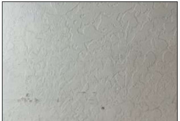
12: Heavy Trowelled Drywall System Sample ID: 005-34-36
