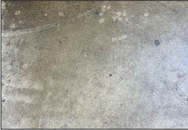
13: Exterior Concrete Sample ID: 005-37-39
