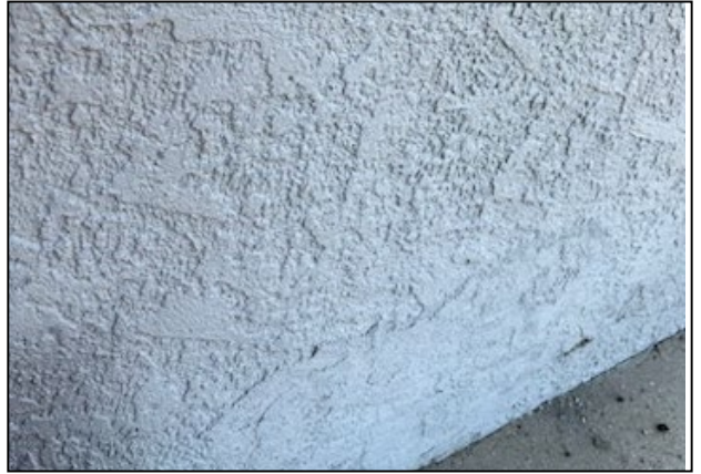
14: Exterior Stucco Sample ID:005-40-42
