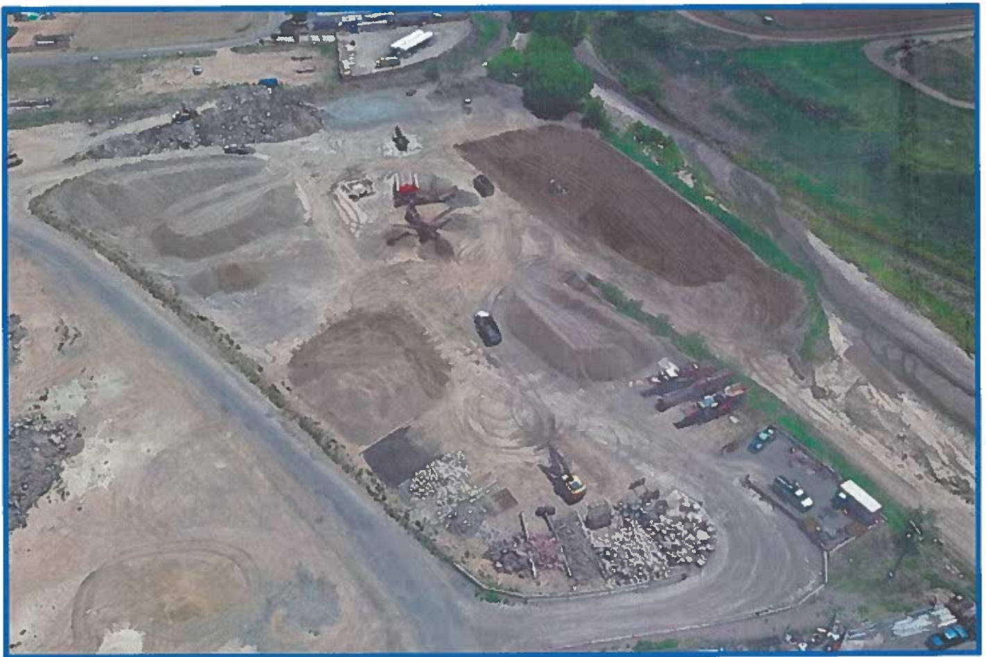
Earth Resources Corporation crushing & screening operations area
