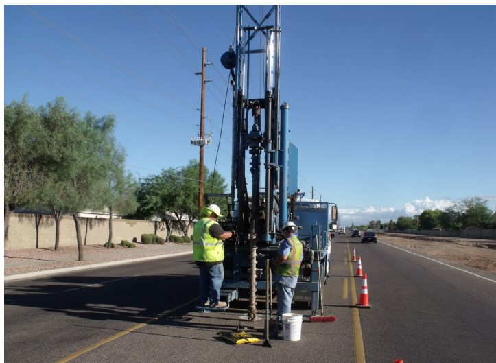
Geotechnical Roadway Drilling
