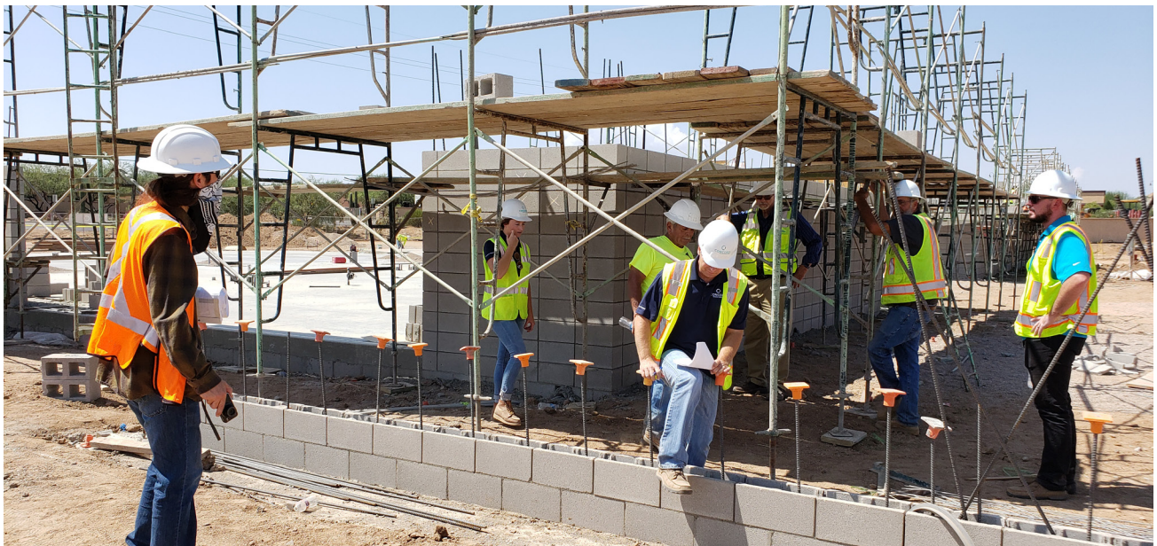
Above: Line and Space conducts regular jobsite visits to check construction progress and contractor compliance with the Construction Documents.
