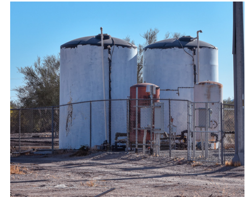
Existing Water Infrastructure
