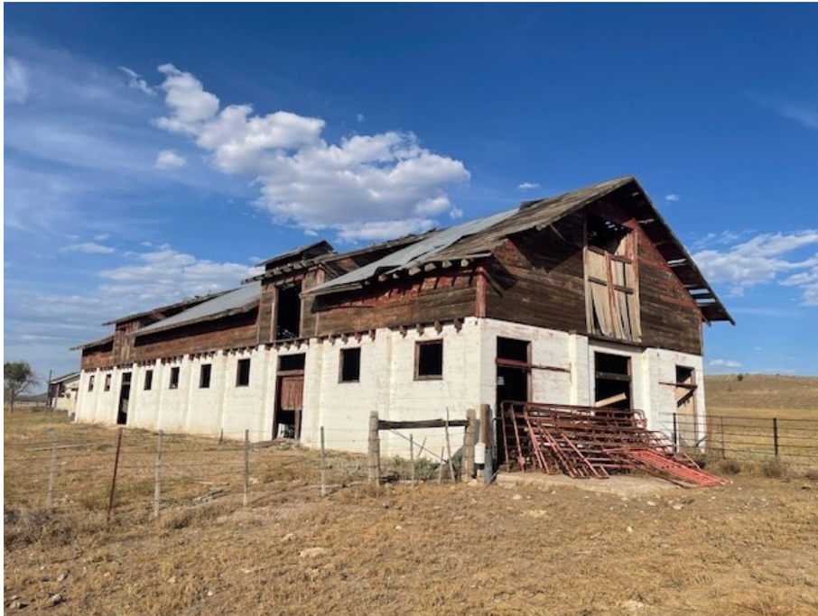
View of southwest corner.
