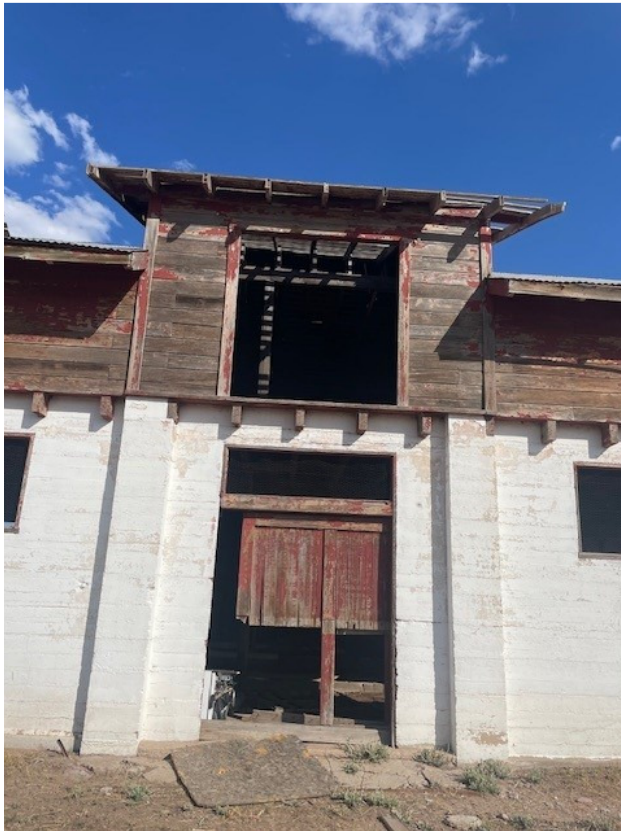
Typical exterior condition.
