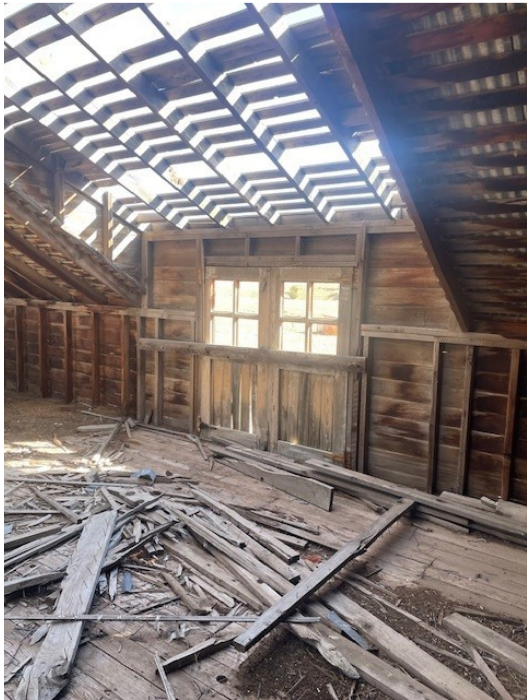
Typical condition of hay loft.
