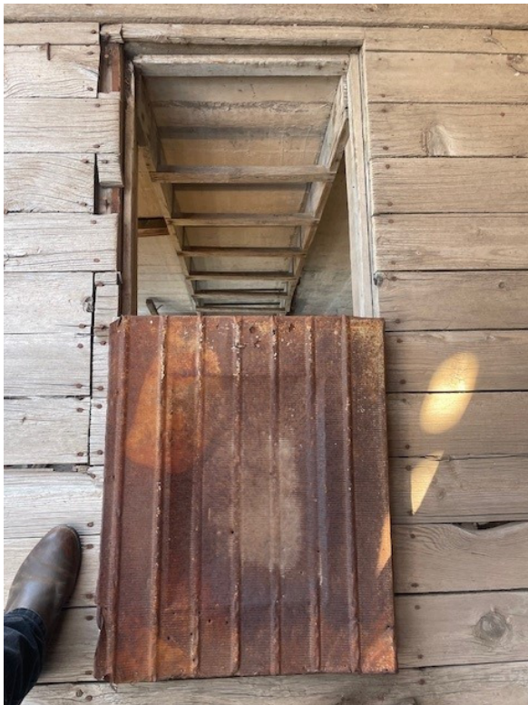
Hay loft access hatch showing original metal ceiling panels to keep milling space clean.
