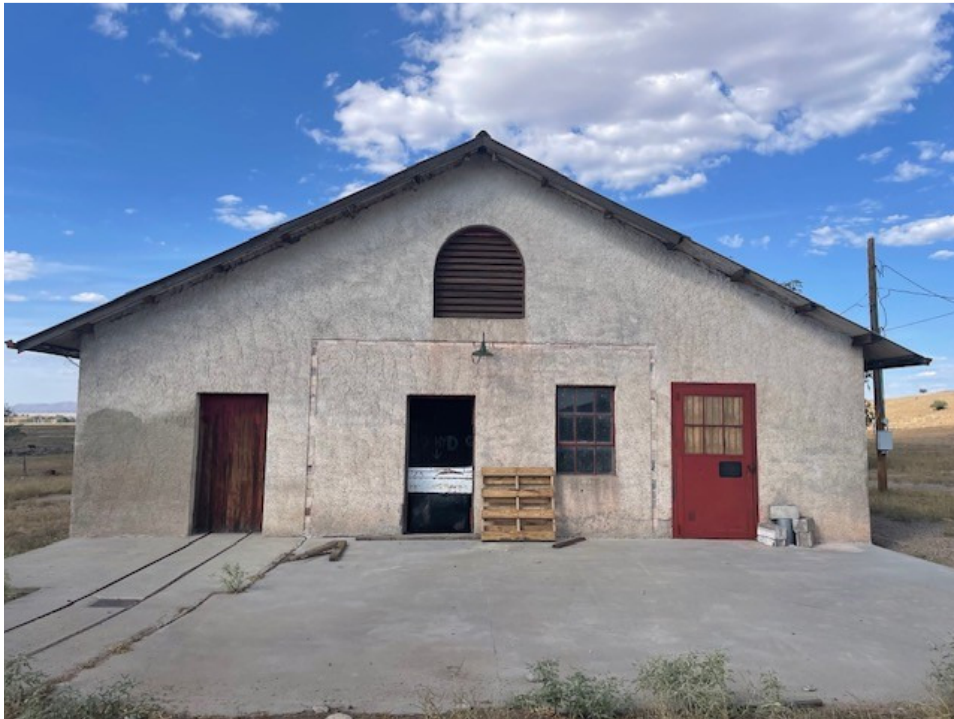
South elevation, showing track from dairy barn. Gunite stucco finish on poured In place concrete walls.
