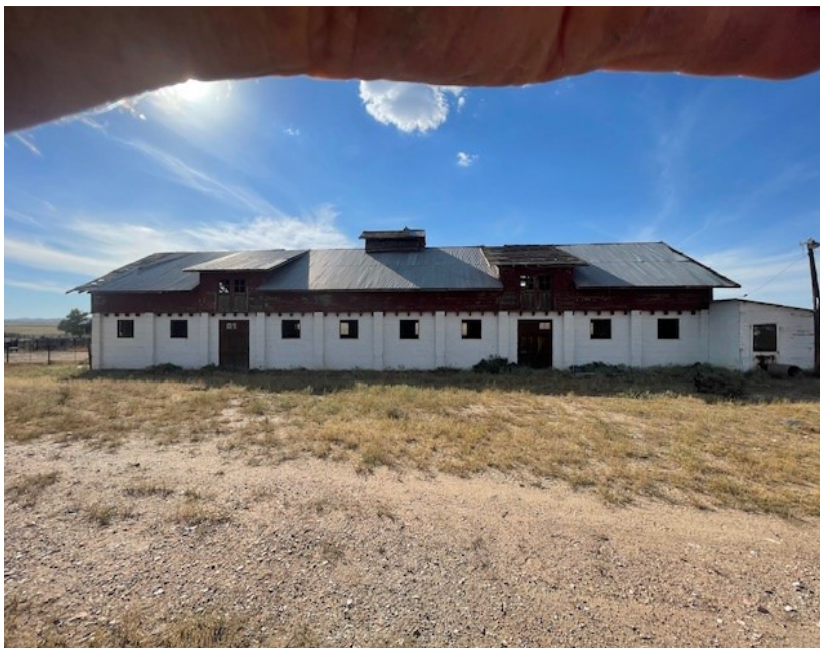
East elevation, paint doors, cover windows with OSB.
