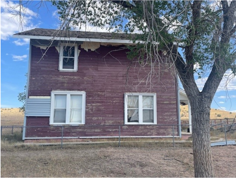
West elevation. Remove nails, prep, prime and paint siding.
