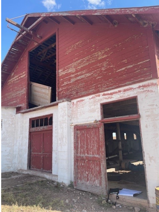
Partial north elevation.
