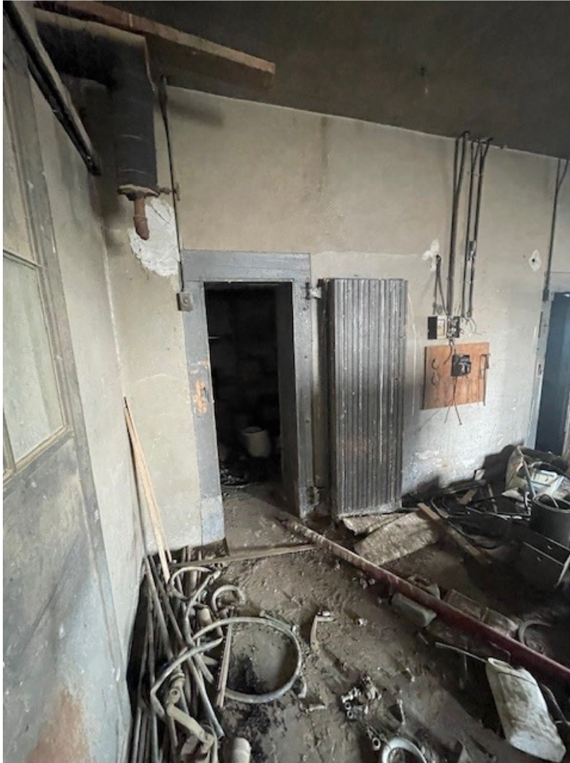
Door in cold storage room.
