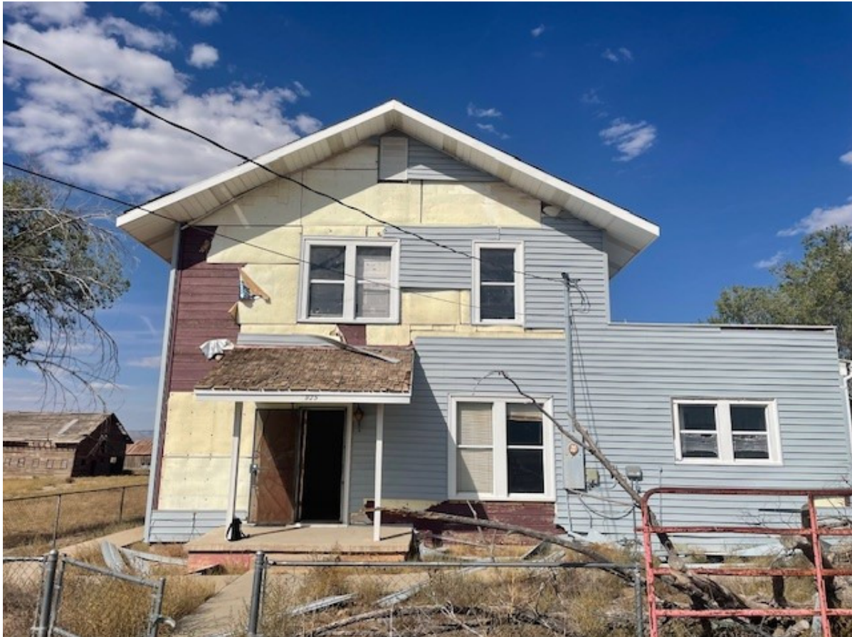
South elevation, remove remaining vinyl siding, foam and nails.
