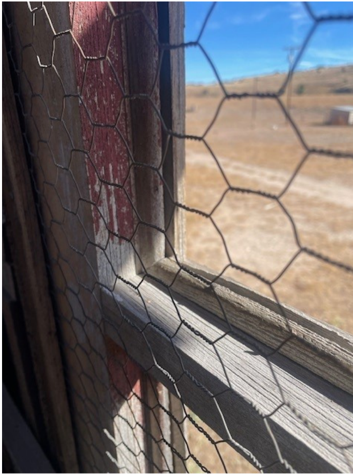
Hayloft window, originally glazed, covered with chicken wire.
