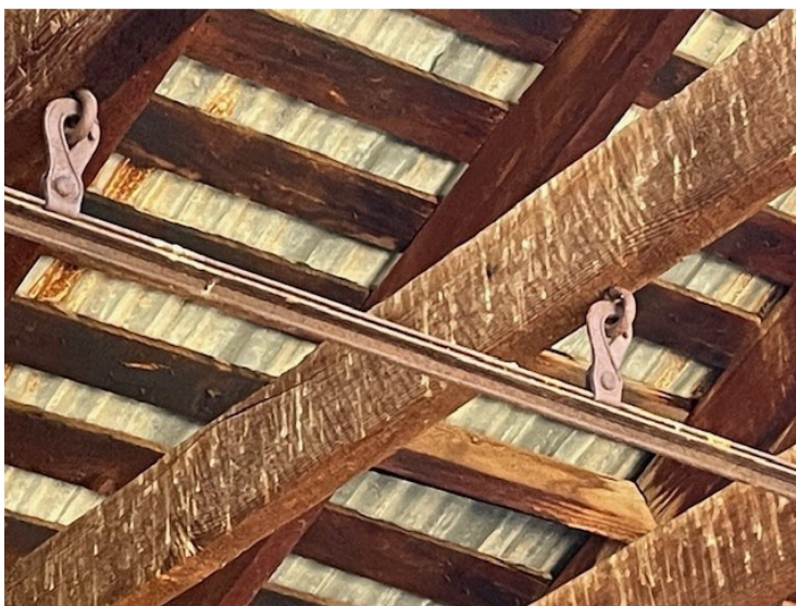
Hay bale transport track at cross tie in hayloft roof.
