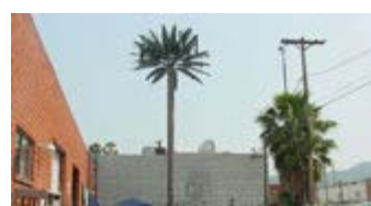
▣ Figure 9 Tower Camouflaged as Palm Tree
