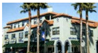
▣ Figure 5 Tower Disguised as Chimney
