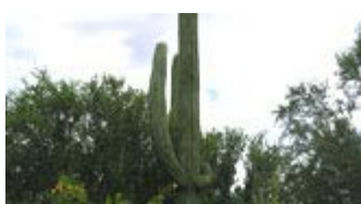
▣ Figure 10 Tower Camouflaged as Cactus
