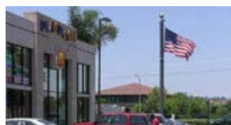
▣ Figure 6 Tower Disguised as Flag Pole
