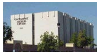
Figure 3 Representative Facade Mounted Antennae
