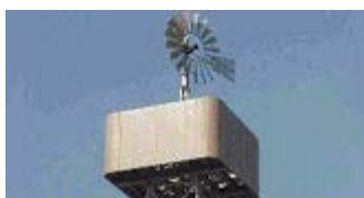
▣ Figure 11 Tower Camouflaged as Windmill
