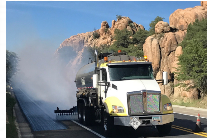
Applying PMAR Binder for the City of Prescott SR 89 PMAR Chip Seal
