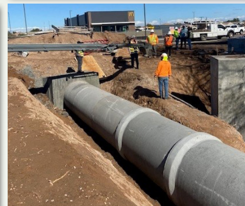
Crews working to complete Salt River Project (SRP) Irrigation Improvements at Avondale Blvd and Lower Buckeye Road, February 2023
