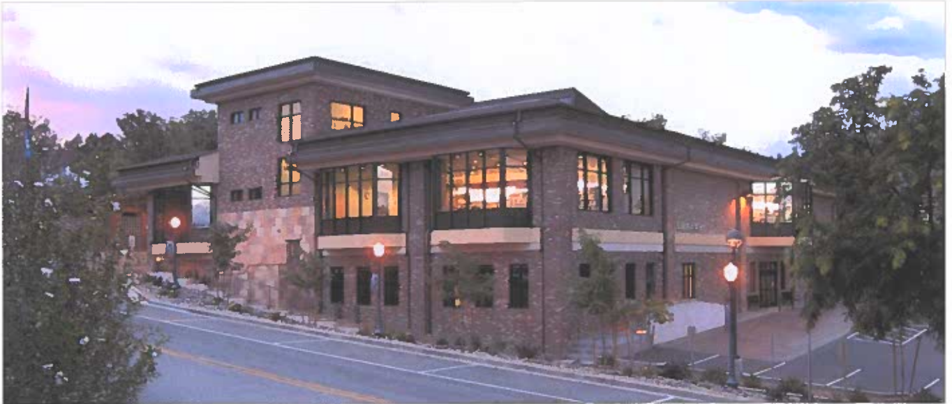
Prescott Public Library Renovation & Expansion; Prescott, Arizona; 38,892 SF
