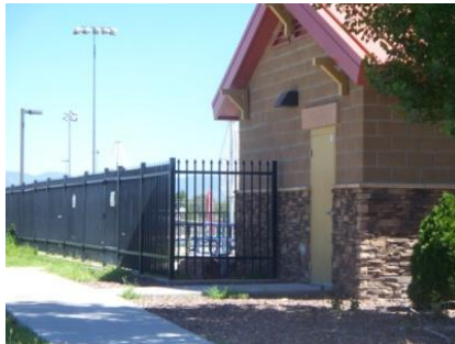
North end of building – add fencing to secure north ingress-egress
