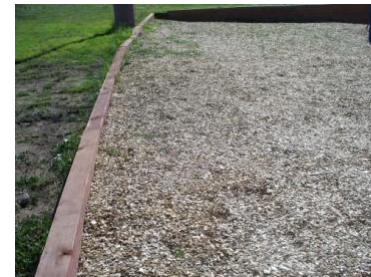
Desired engineered wood fiber (a.k.a. Fibar) and borders (i.e., treated lumber or composite)
